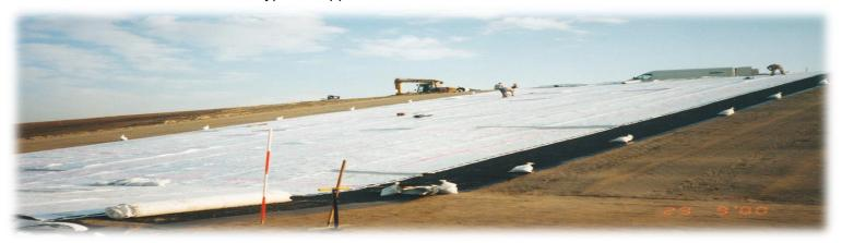
Roads RE Wall, Levelling and mechanical protection of the geomembrane; drainage of the accidental leaks below primary; leachate and rain water collection above primary geomembrane; mechanical protection of the geomembranes when in contact with wastematerials and/or soil; drainage of liquids and gases present in the soil above and/or below the capping geomembrane.
